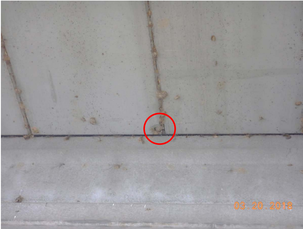
Photo 1: Element 8098: Showing spall with exposed steel Panel 8 in Bay 1-1
