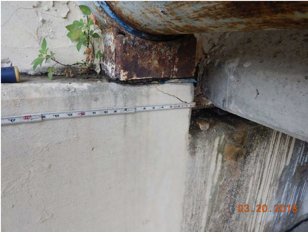
Photo 5: Element 215: Showing delamination at top edge of Abutment 1 Cap.
