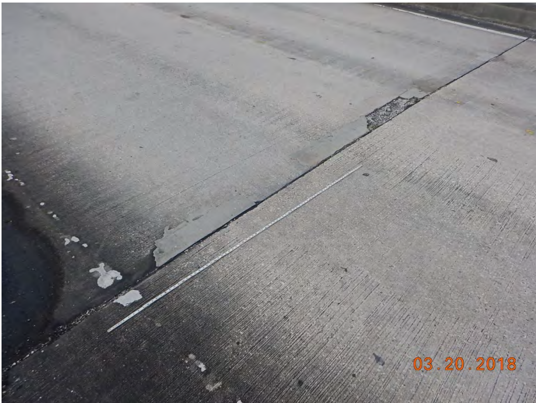
Photo 4: Element 301: Showing spalled area at Bent 3 joint.
