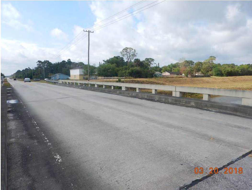
Photo 9: Inspection Notes: Heavily chipped and worn deck striping.
