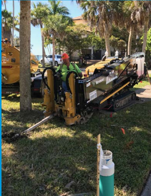
Horizontal or directional boring equipment
