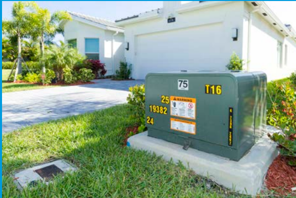
Pad-mounted transformer
