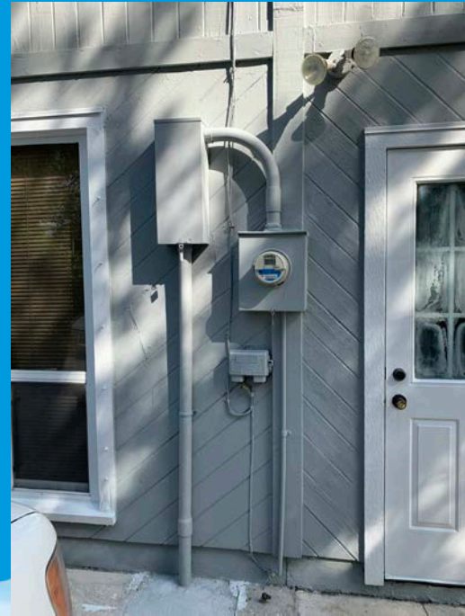
Meter enclosure adapter box connected to meter enclosure
